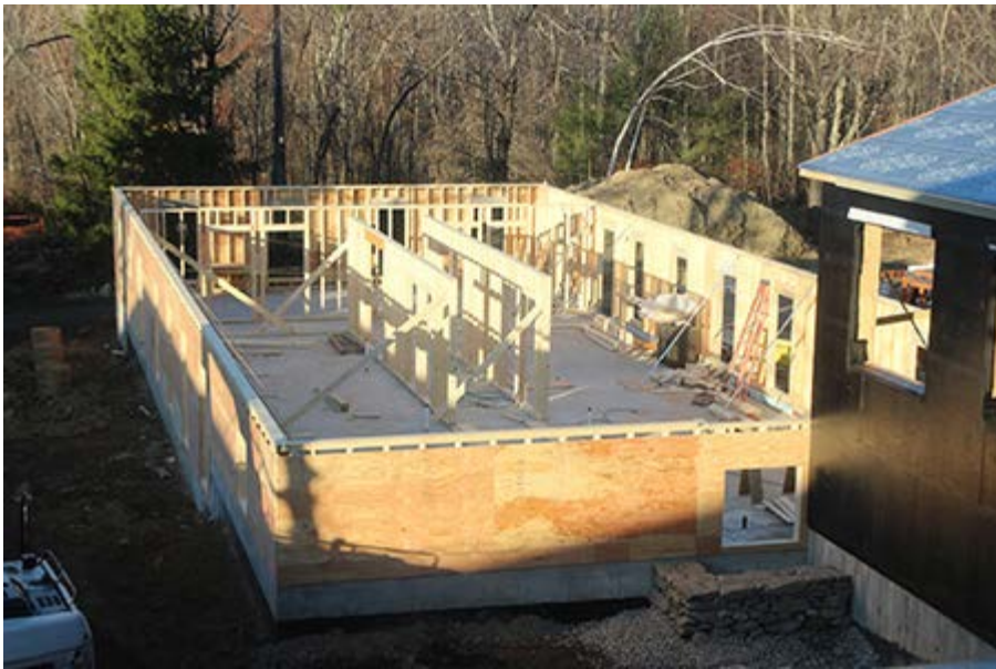
The framing for the first floor of the new dormitory.
