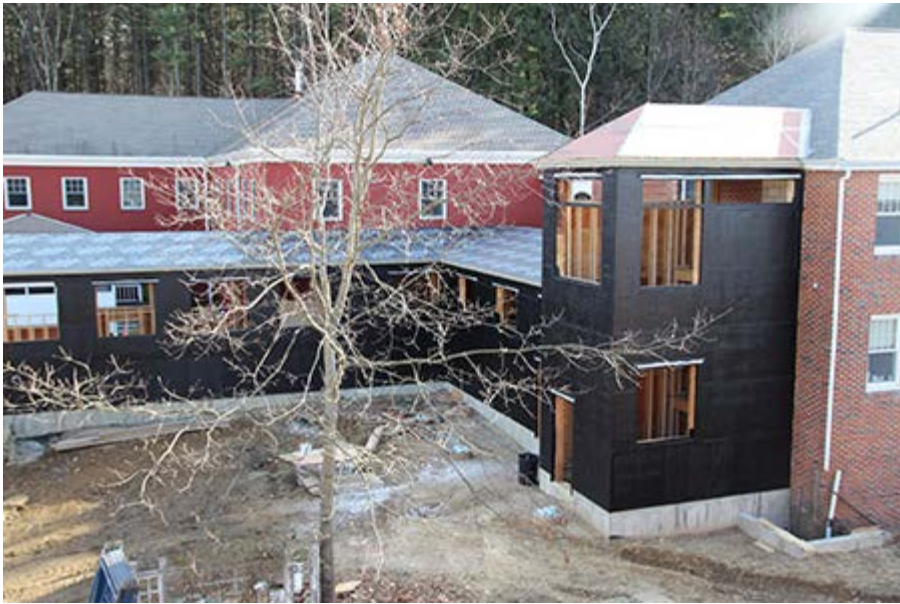
Construction proceeds apace on the connector and stair tower.
